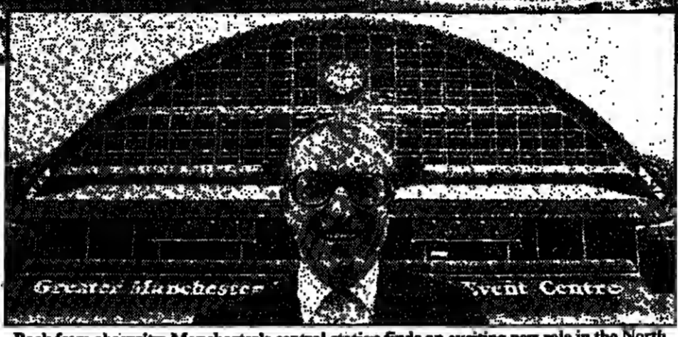
Back from obscurity: Manchester's central station finds an exciting new role in the North West's transformation as the G-MEX exhibition centre with Frank Winter at the helm.
